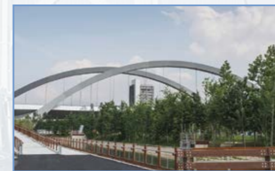
Expo Bridge, Milan (Innoventions)
